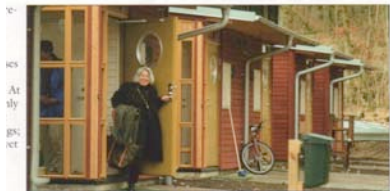
● External walls are exceptionally well insulated and airtight. A glazed porch protects the entrance door.
